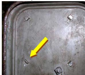
These tabs did not bend easily (lower left). Would they survive bending back down to re-secure the
